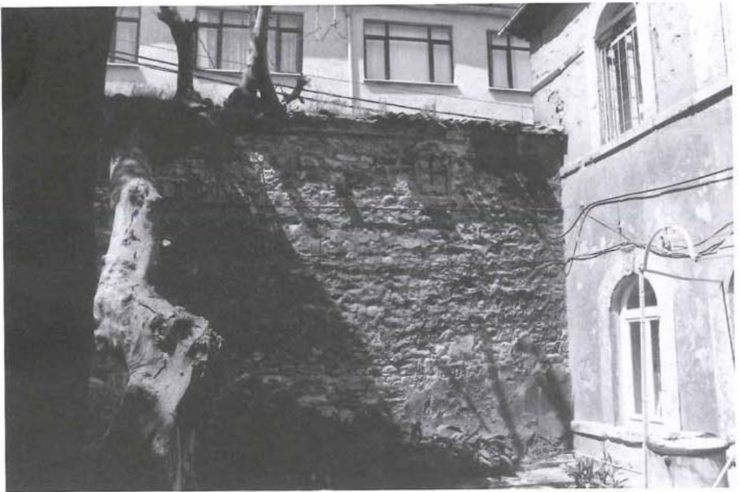
Plate 40 Church of Saint George terrace wall
